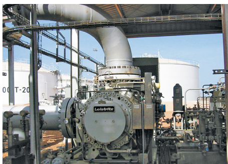
Dual mechanical seal EagleBurgmann SHV-D4/170-E1 installed at Exxon Mobil in Chad (Africa) in a Leistritz twin screw multiphase pump. Operating conditions: t = 54\text{ °C} ( 129\text{ °F} ), p = 30\text{ bar} ( 435\text{ PSI} ), n = 1,200\text{ min}^{-1} .
