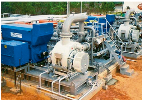
Single mechanical seal EagleBurgmann HSHJ42S6/80-E1 installed at Ameriven (Venezuela) in a Bornemann twin screw multiphase pump. Operating conditions: t = 38\text{ °C} ( 100\text{ °F} ), p = 8\text{ bar} ( 116\text{ PSI} ), n = 1,800\text{ min}^{-1} .
